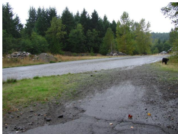
Figure 5 Cement haul road
